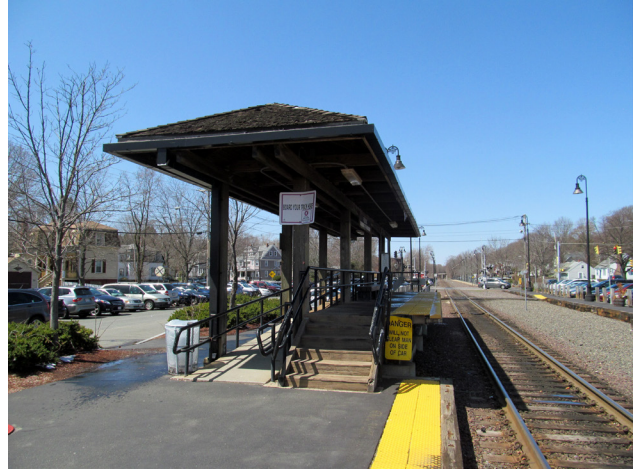
A mini-high platform, seen here at Reading, provides an easier boarding experience than a low-level platform on its own, but still reduces the rate at which people can board.
