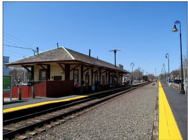
Despite having two platforms, the current Reading station only has a single track. Moving the station slightly south removes the need to build a second track, and helps avoid several nearby grade crossings.
